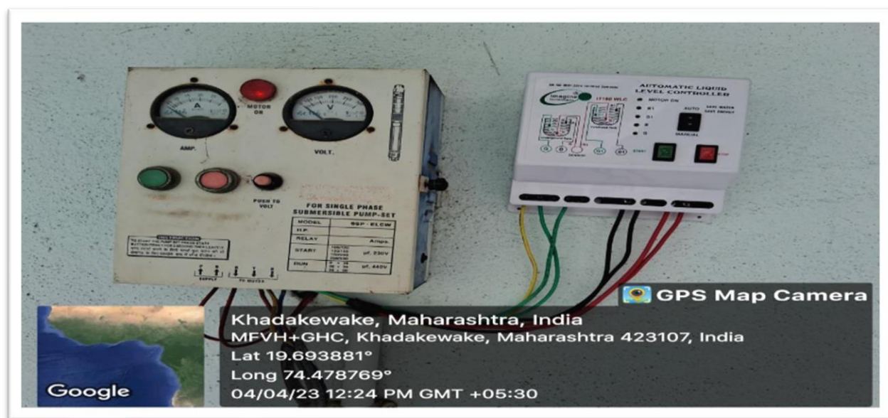
Photo 1: Sensor based Automatic Water Level Controller
